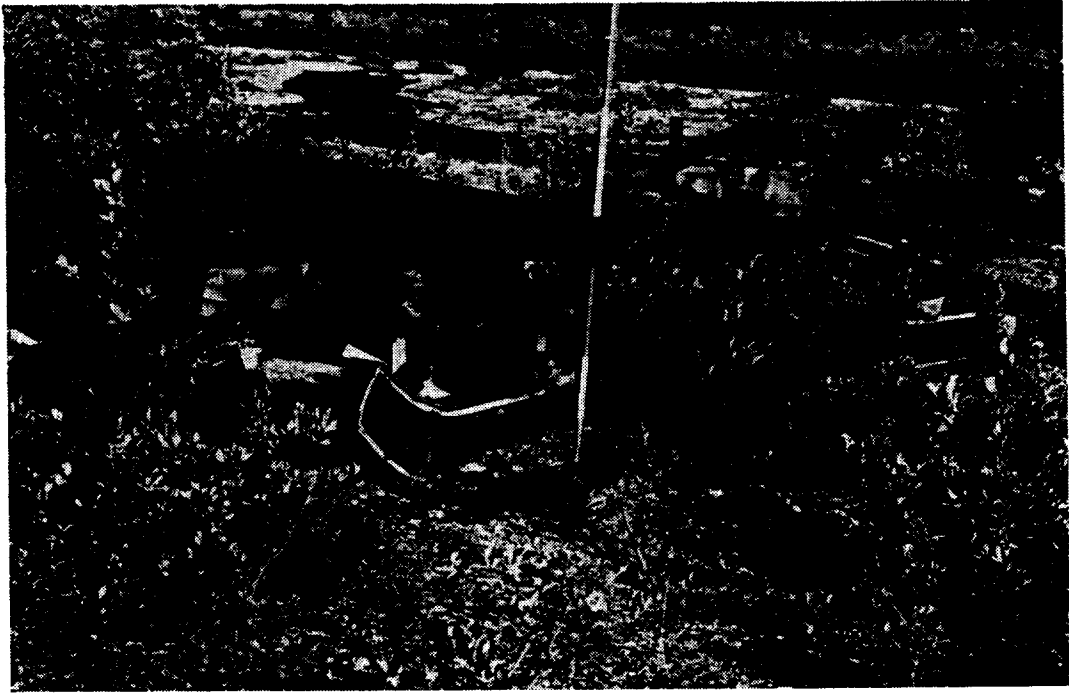
Plate 3.10 Sleds such as this were dragged behind bulldozers. They carried any of the heavy freight such as pipe, power plants and welding machinery (photo by Kershaw 1977).
