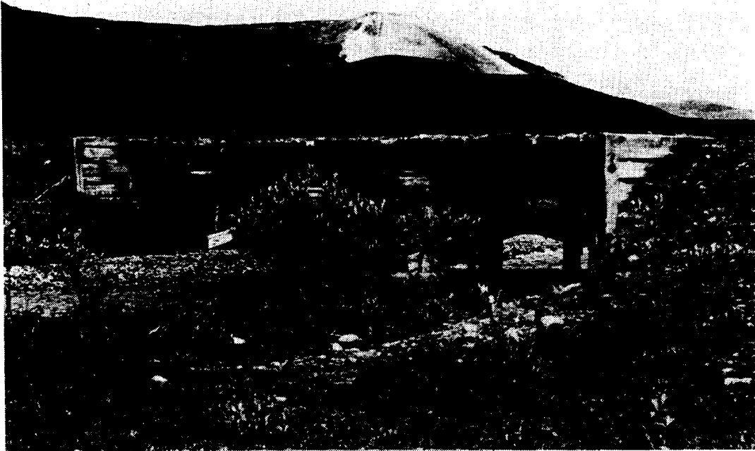
Plate 3.15 Other bridges, such as this one at Mile Post 207.5E are in very good condition (photo by Kershaw 1979).
