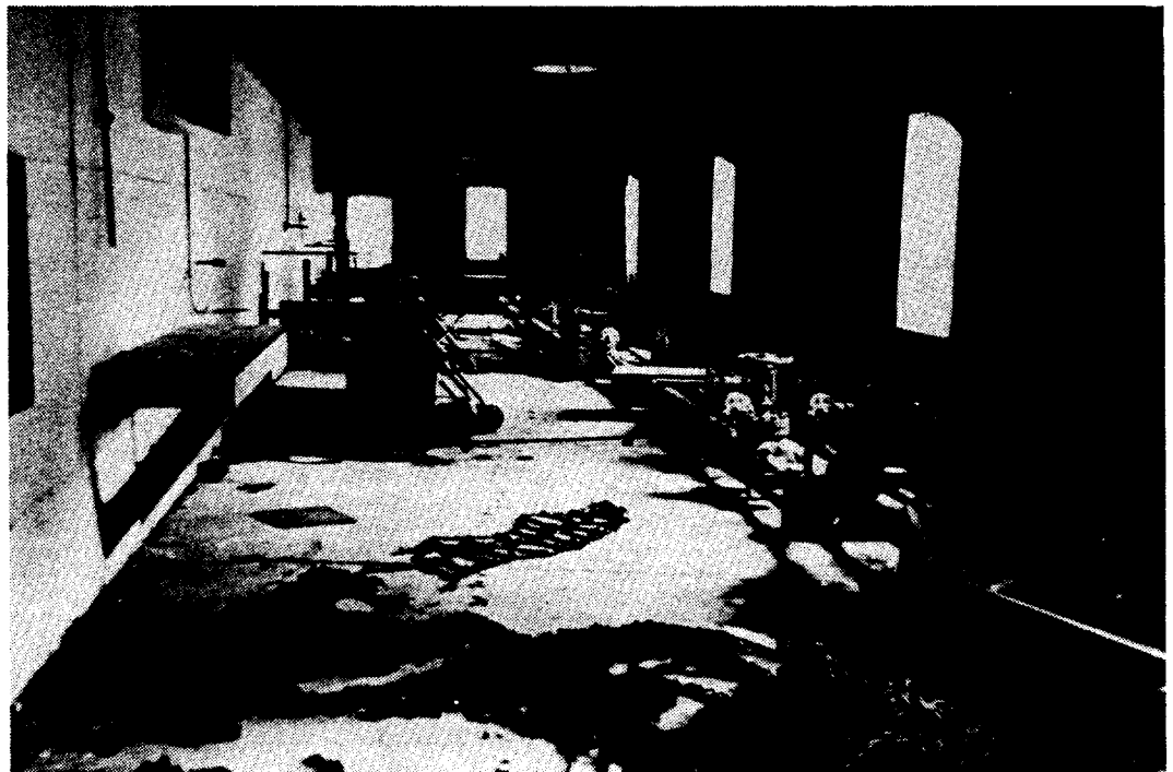
Plate 3.6 The pumphouse at Station No. 2 has many of the pipes but the pumps have been removed. This is similar to the situation at other pumphouses. Tire chains litter the cement floor (photo by Kershaw 1977).
