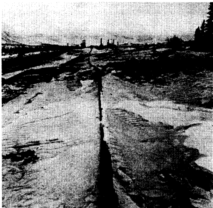
Plate 1.5 The completed CANOL No. 1 pipeline was above-ground and often close to the tote road (photo by R.S. Finnie).
