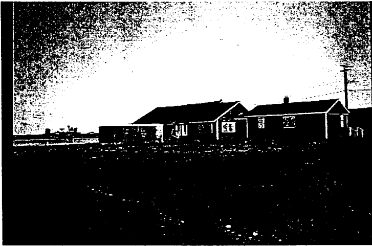
9. North View of Old Furshop Building
