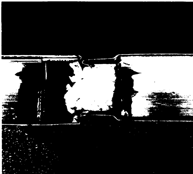
Fig. 5.3 Prefabricated aluminum-panel joint detail
