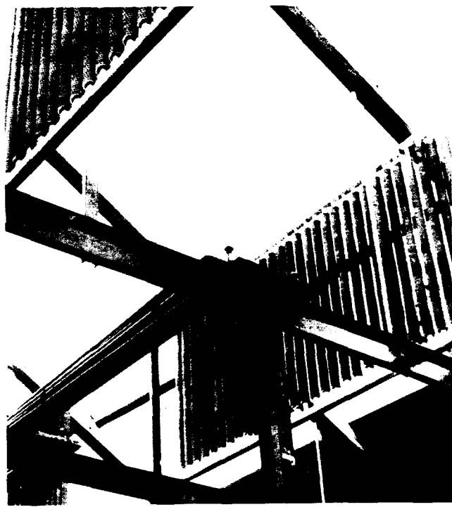
Fig. 5.11 Finned-pipe radiators in place during construction
