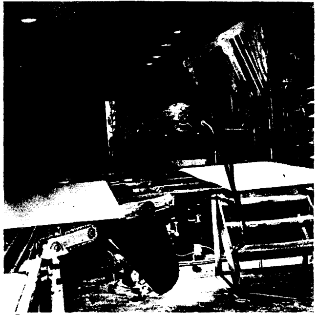
2 The 10-opening press has demanded cauls; the side-shift mechanism has responded. Feed belts on main conveyor drop, allowing rubber rolls to shift cauls obliquely and deliver them to feed belts serving elevator.
