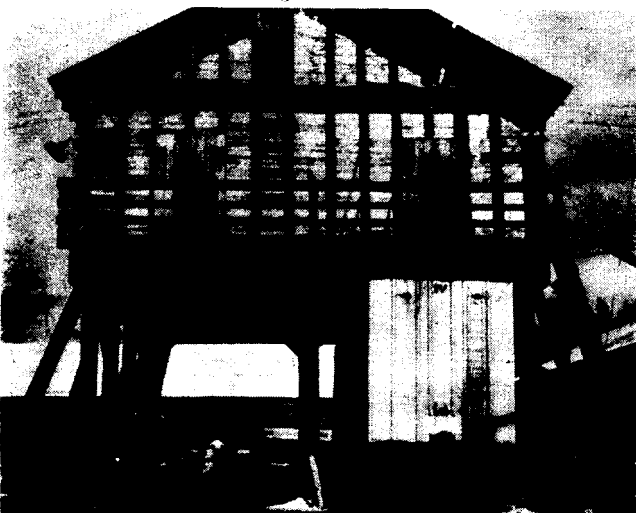
Chip bunker loads Utility trailer. Company trucks haul fir chips to U. S. Plywood, Lebanon, Ore., for hardboard production, and hemlock chips to Crown Zellerbach.
