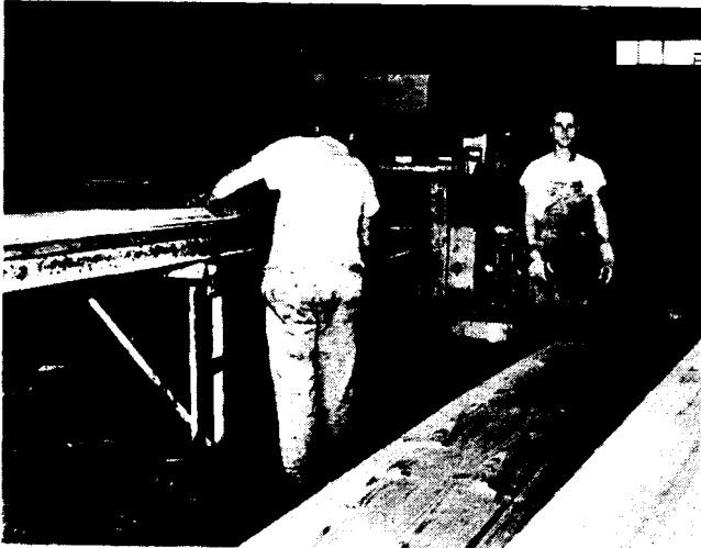
Lumber surfaced on two sides is first run through the glue spreader and laid up to proper thickness on a jig-table. Two men handle gluing and two on layup.
