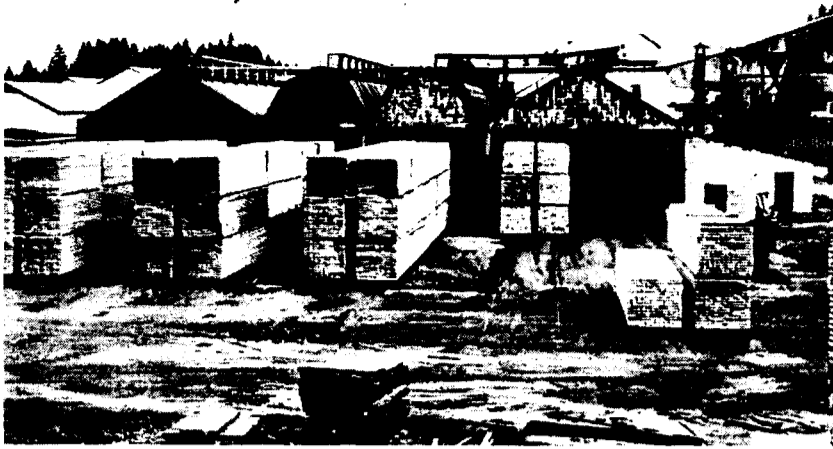
Product refinement for A. J. Frank consists of drying and surfacing all stock. Moore 66' oil-fired kilns are two double and two single units at left. Residue utilization is
