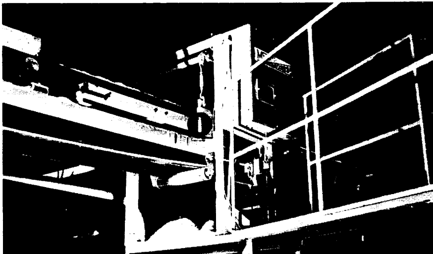
This is how the weighing mechanism was installed on the conveyor belt. Circle marks one of the rollers on which the belt rides. Rollers are mounted in the framework ( I ) which is suspended so that weight variations are sensed continuously and recorded.
