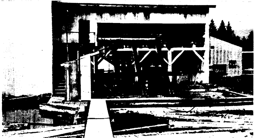
kicked back "into pond automatically. 'Logs" enter mill through sidelift at right. Logs from 12' to 26' long processed in two sorts-60" to 18" and 19" to 35".
