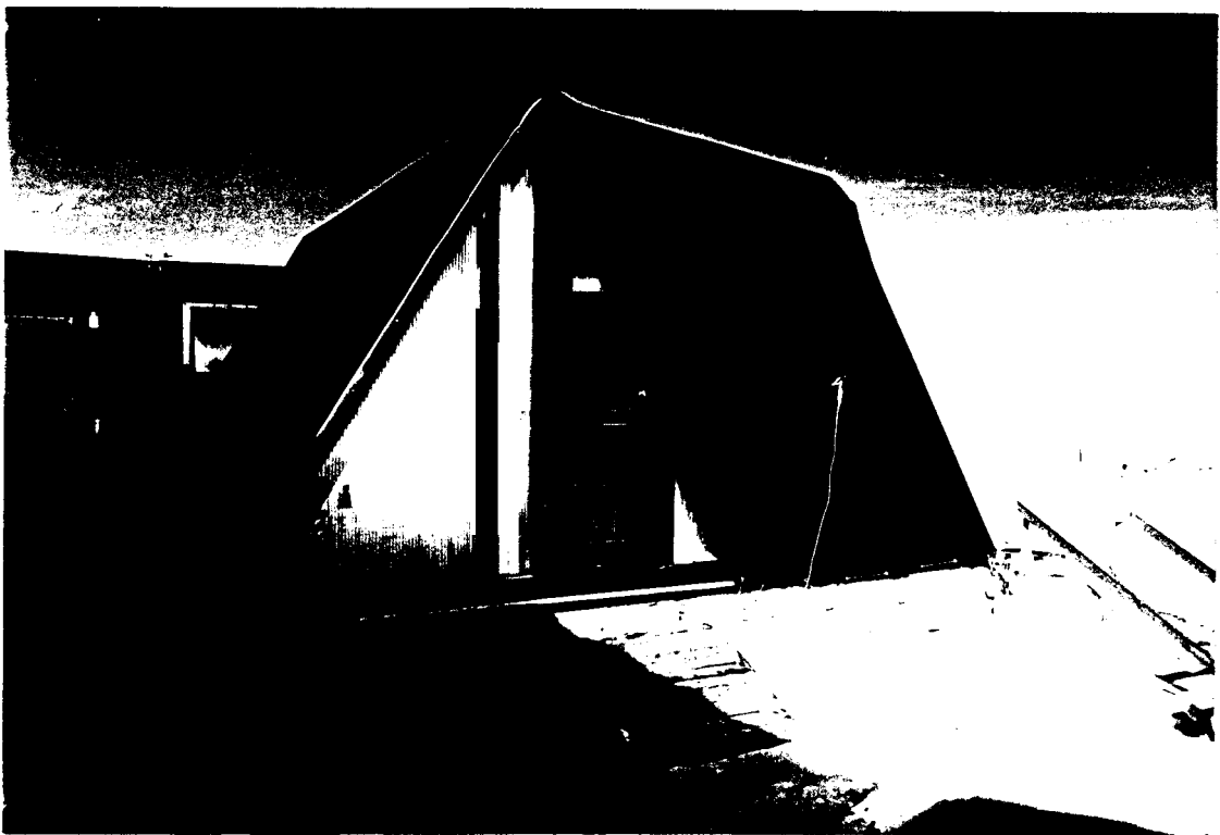
PHOTO 4 : The relocated greenhouse structure following the completion of construction Phase 2. May, 1986. Greenhouse is mounted on heat storage foundation and is fitted with canvas cover and insulation.
