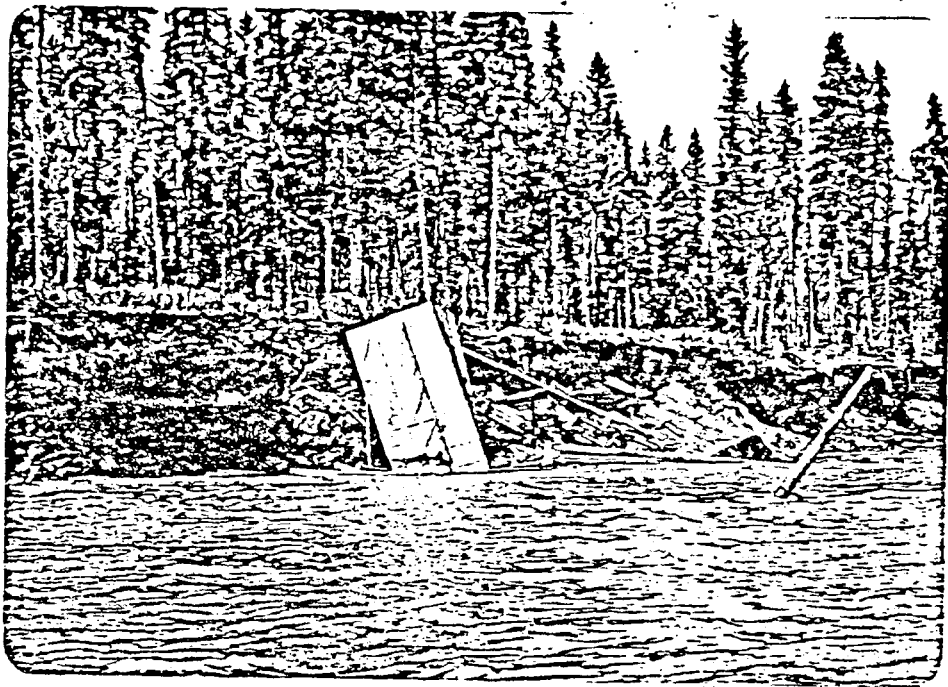
Figure 13.1 One of the hazards of building next to the river. In 1968 these cabins were 18 m from the river edge and in 1974 they are obliterated.
