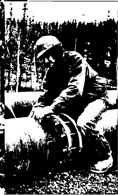
▲ Tailing line maintenance, Colomac Mine.
