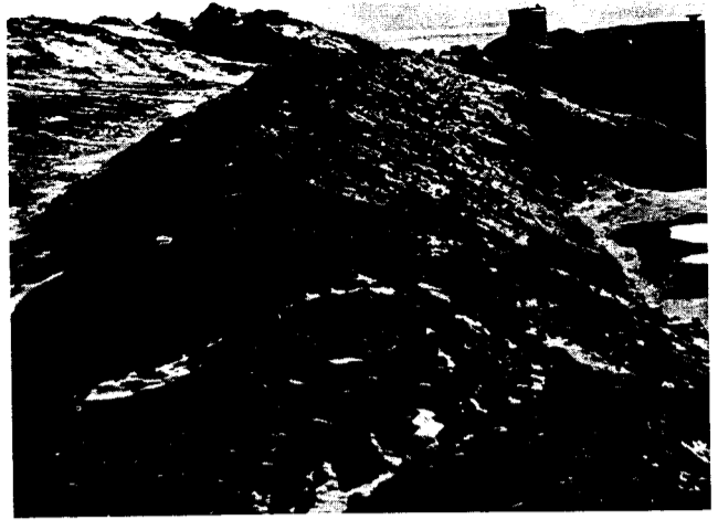
Berms can provide drainage in permafrost areas
