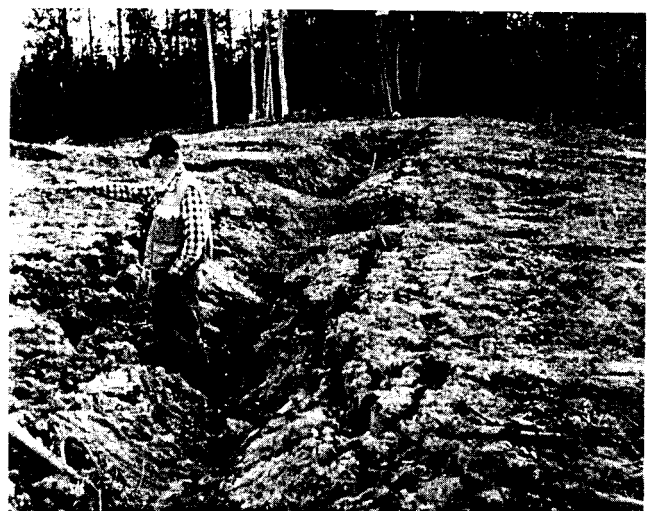
Failure to compact backfill material can result in post-abandonment subsidence
