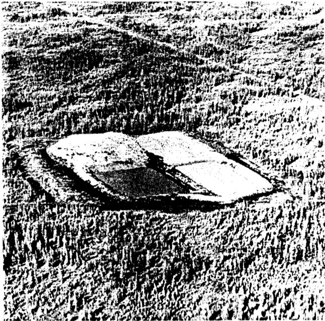
Drilling conditions sometimes necessitate construction of a supplementary sump
