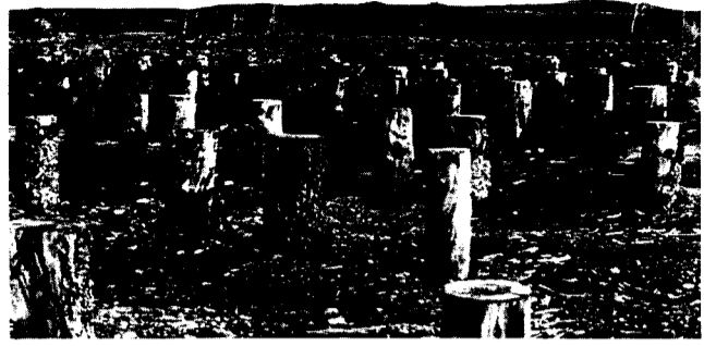
Granular pad subsidence can expose abandoned piling butts
