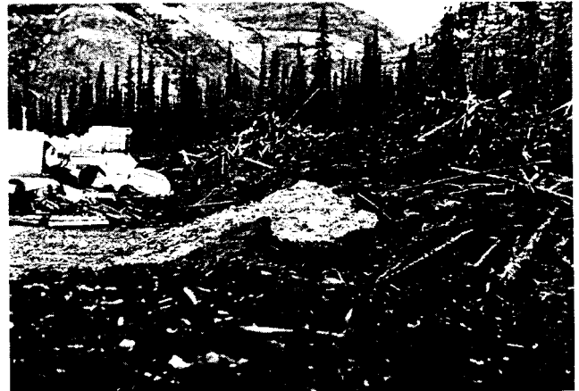
Windrow timber cover at the well-site edge
