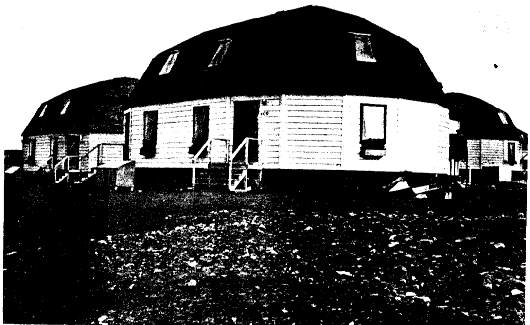
The mining company carried out some experiments in their housing program. Their duplexes are elliptical and with domeshaped upper floors. The houses were said to be expensive and difficult to furnish.
