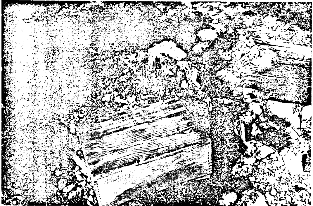
Plate 3.18 Even after 39 years this dynamite box still retains the warning instructions. Up to 20 sticks were employed to blast holes in bedrock and frozen ground for telephone poles (photo by Kershaw 1978).
