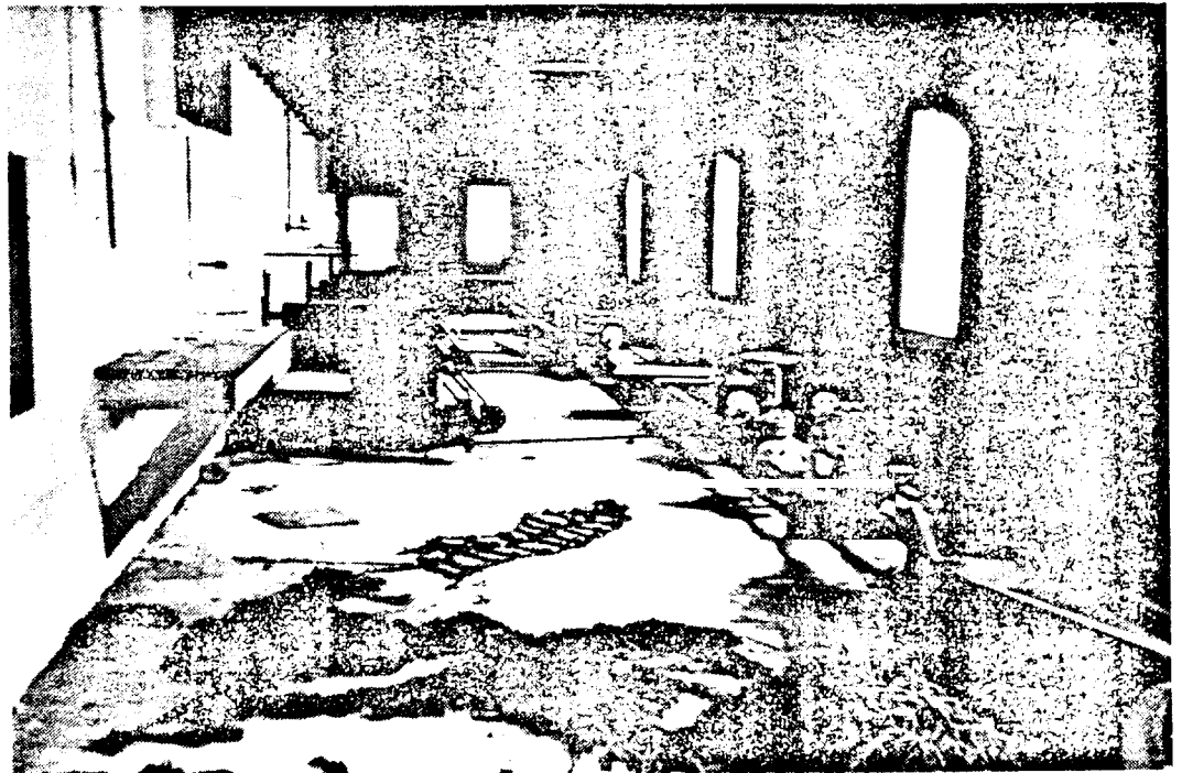
Plate 3.6 The pumphouse at Station No. 2 has many of the pipes but the pumps have been removed. This is similar to the situation at other pumphouses. Tire chains litter the cement floor (photo by Kershaw 1977).
