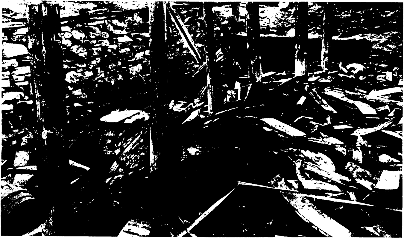
Figure 6 The disturbed interior of Kellest's storehouse, as photographed in 1977. The dark mass in the centre of the photograph is coal.
