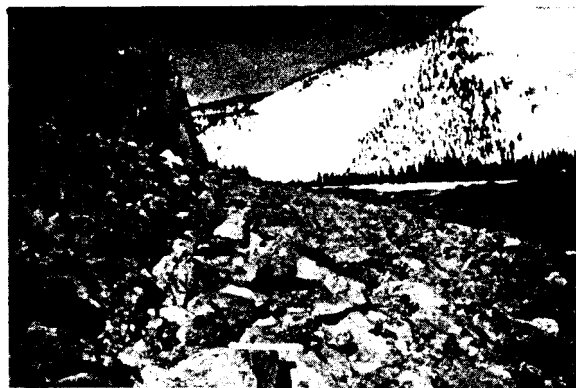
• rip rap used for bank protection
