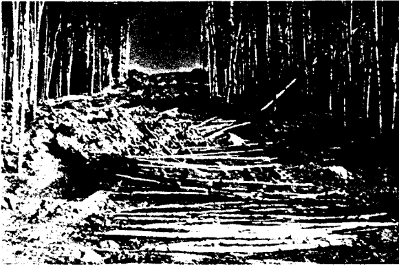
. slash used to reduce further erosion
