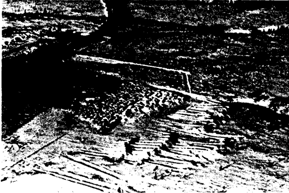
. overburden and topsoil removed separately
