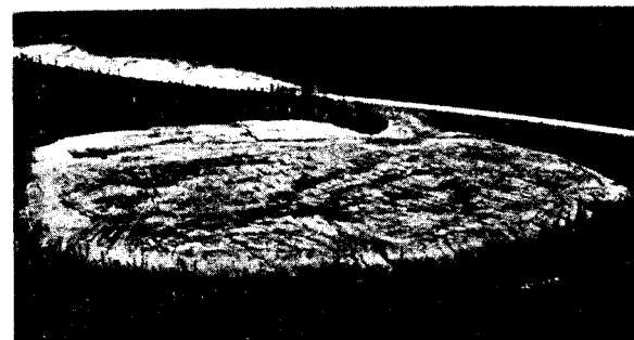
• removal of overburden to a natural depression • overburden spread and contoured to low profile x do not smother well vegetated ground
