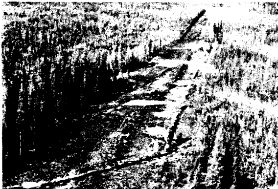
.the opening in the berm allows cross flow on this right-of-way
