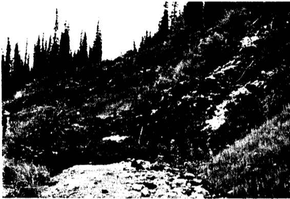
reclamation would have prevented this slumping
