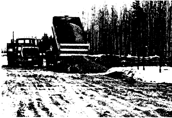
.backfill with thaw-stable (ice-poor) soil
