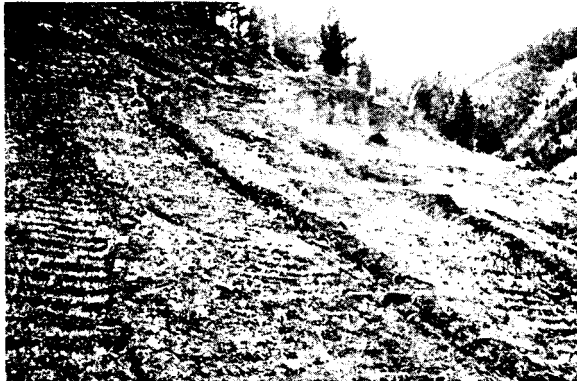
.cleat marks from a cat provide microsites for seeds to establish
