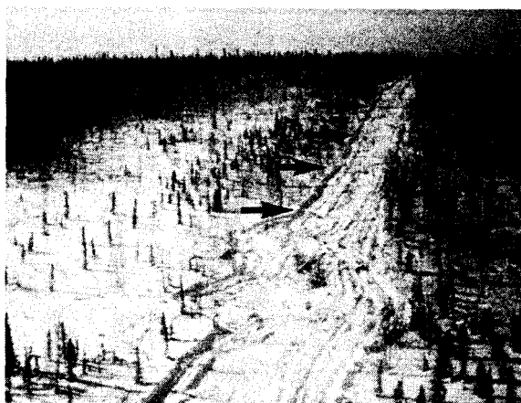
• construction of snow berms and timber roll back will protect this slope from erosion
