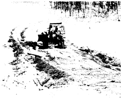
•constructing a snow-filled crossing
