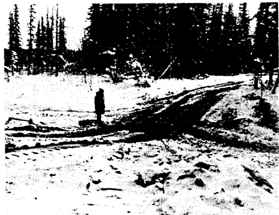
•the use of soil to cap a snow fill is an unacceptable practice
