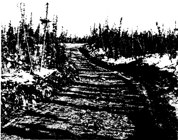
• excessive blading of this access road has removed the snow and surface organic mat and greatly increased erosion potential
