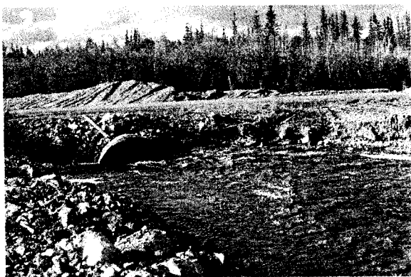
.set culverts into the stream bed to maintain natural stream gradient
