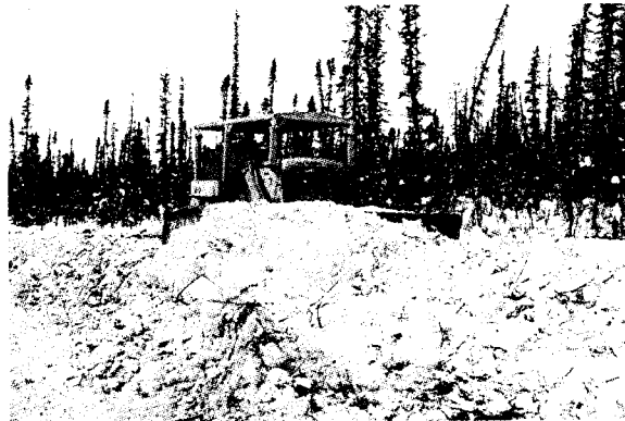
• retain as much snow as possible on the road
