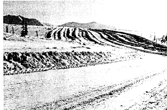
•excessive snow ploughing has created snow banks along the road; these can disrupt natural drainage
