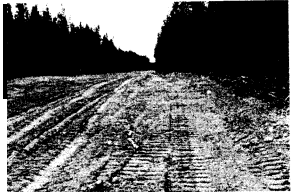
, a cleared right-of-way for a haul road
