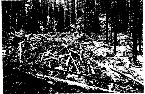
• a right-of-way cleared by walking down the vegetation during winter
