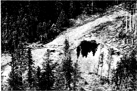
.if drainage is not maintained, road washouts can occur
