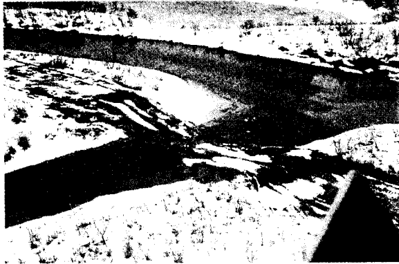
• soil should not have been used in this snow fill
