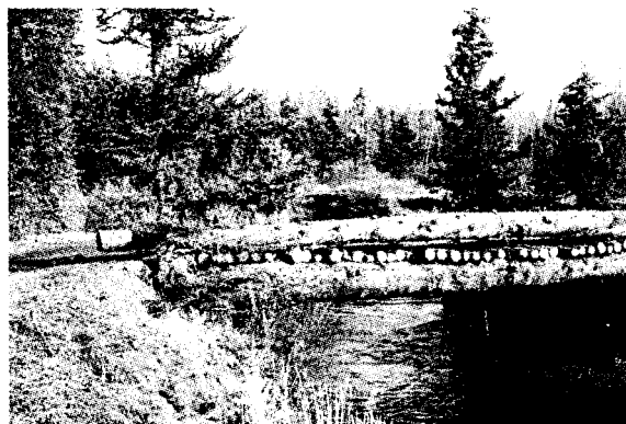
.set culverts into the stream bed to maintain natural stream gradient
