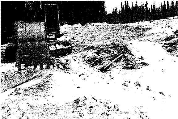
• snow fills and ice bridges must be removed prior to break-up
