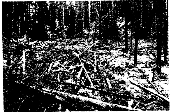
• a right-of-way cleared by walking down the vegetation during winter
