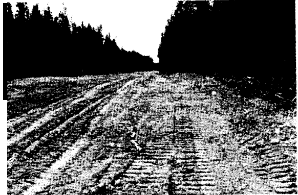
, a cleared right-of-way for a haul road
